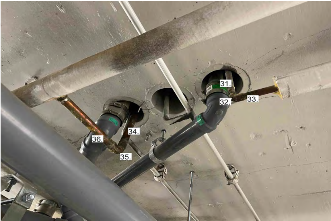
Photograph 6: Middle of Garage Level 1.
