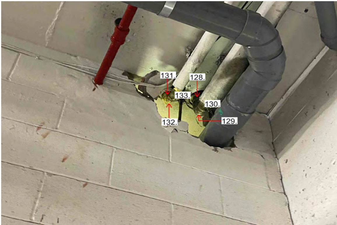
Photograph 23: Parking Garage Level 1A Storage Area.
