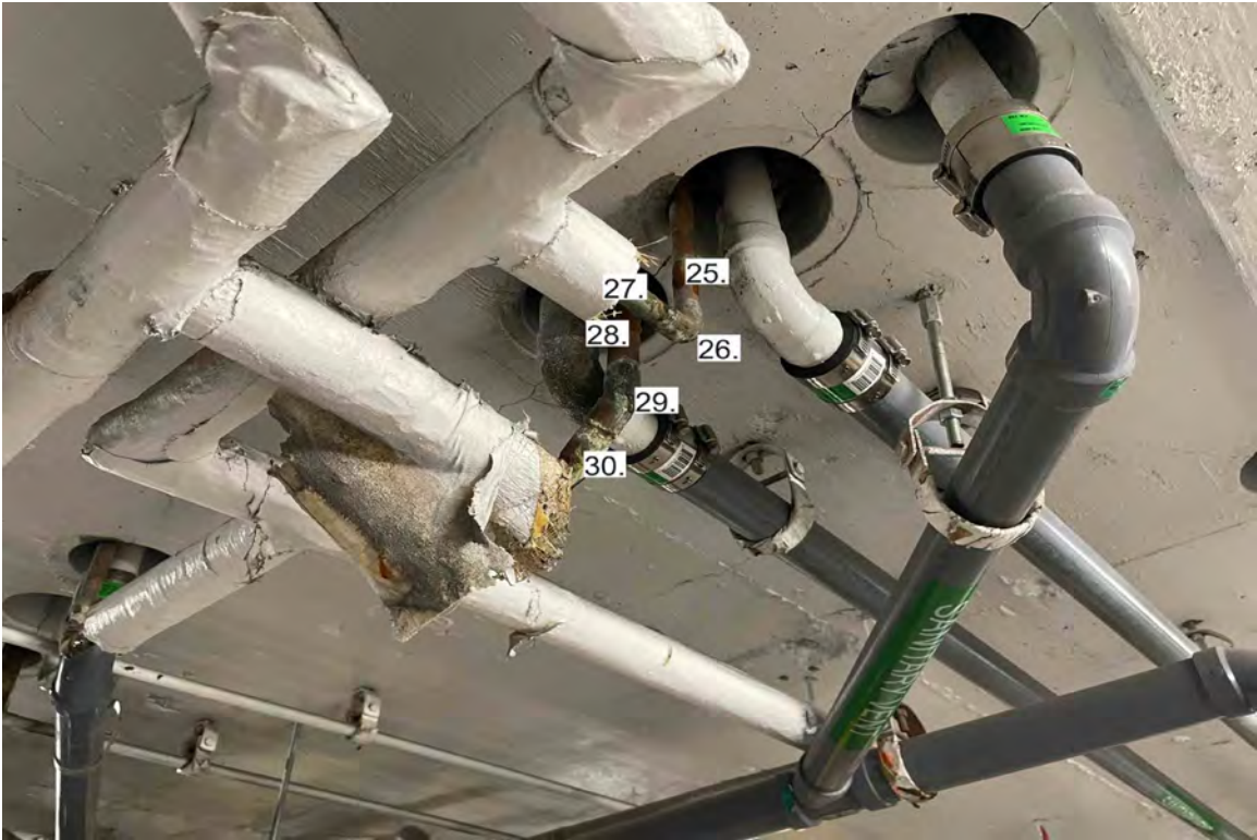
Photograph 5: Middle of Parking Garage by Spot #9.
