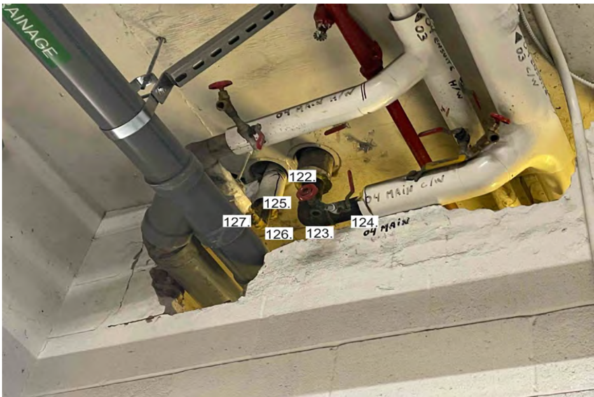
Photograph 22: Parking Garage at Wall across from spot #2 Level 1A.
