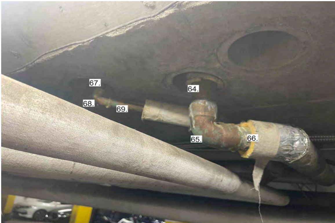
Photograph 12: Near building entrance by spot 33.
