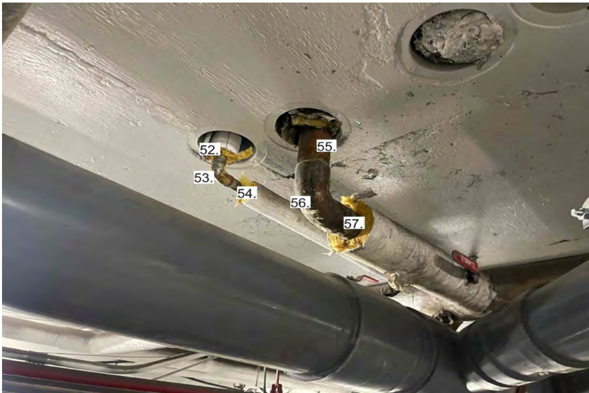
Photograph 10: Outside Generator Room.
