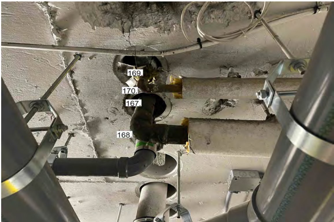
Photograph 32: Parking Garage in front of spot #25.
