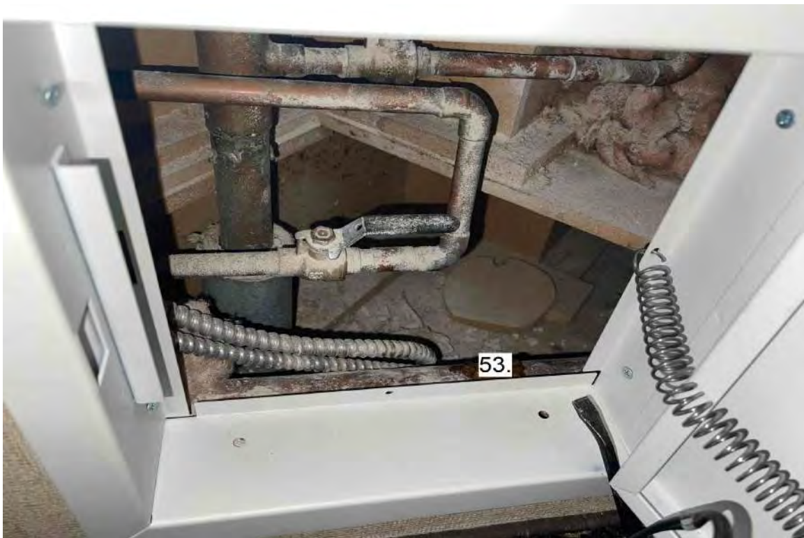
Photograph 28: 6 th Floor Bathroom Stack Unit 610.
