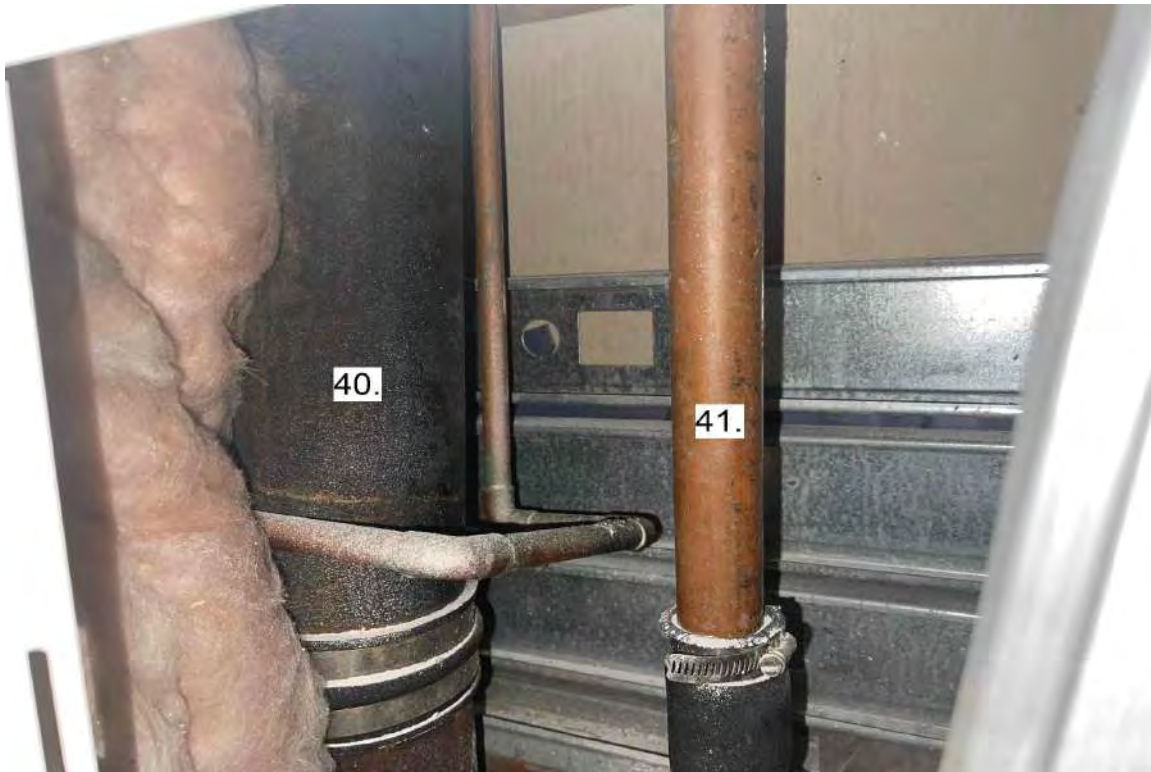
Photograph 21: 7 th Floor Bathroom Stack Unit 706.
