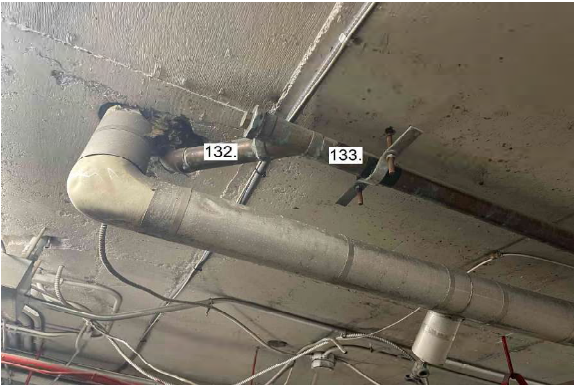
Photograph 39: Level 1 Parking Spot 29.
