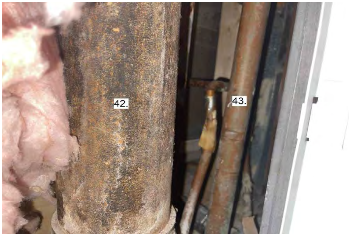
Photograph 22: 7 th Floor Bathroom Stack Unit 701.
