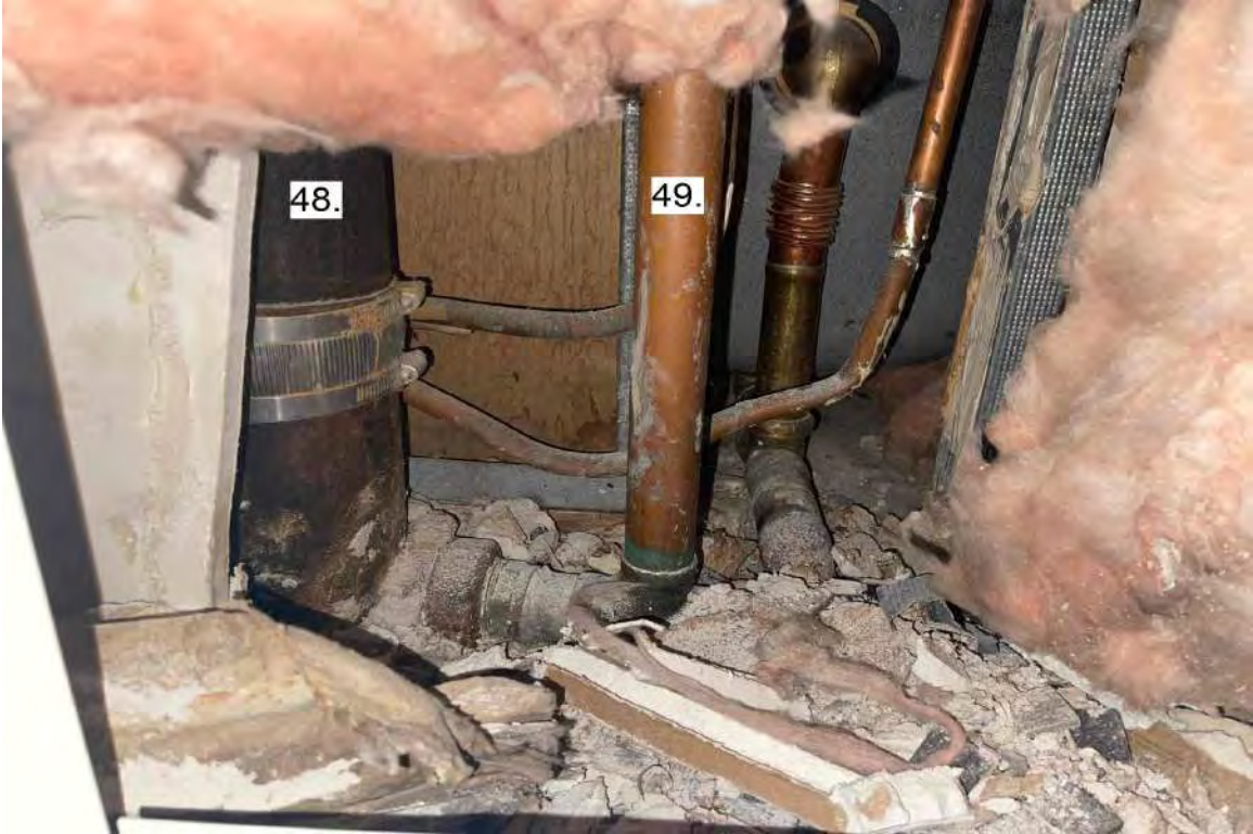
Photograph 25: 6 th Floor Bathroom Stack Unit 606.
