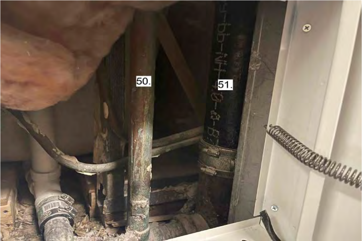
Photograph 26: 6 th Floor Bathroom Stack Unit 601.
