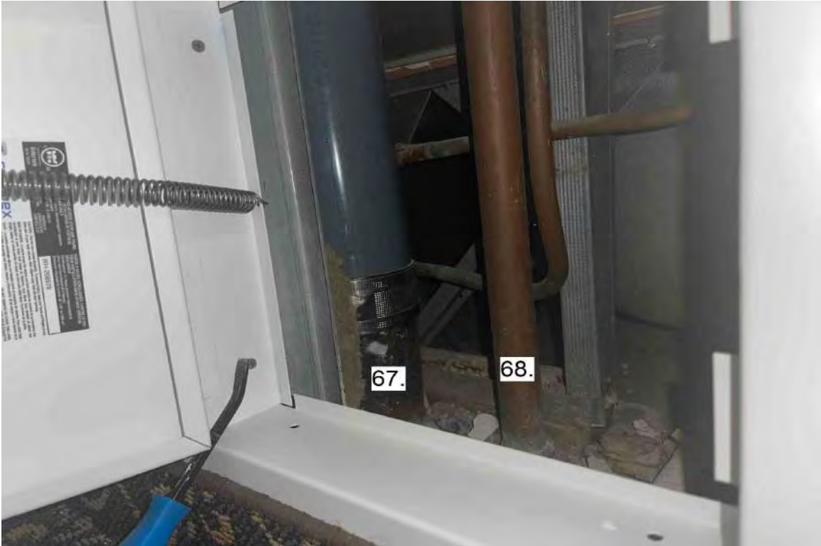
Photograph 35: 4 th Floor Bathroom Stack Unit 410.
