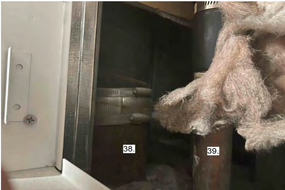
Photograph 20: 8 th Floor Bathroom Stack Unit 807.
