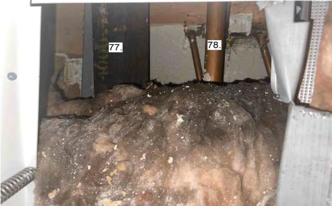
Photograph 41: 2 nd Floor Bathroom Stack Unit 206.
