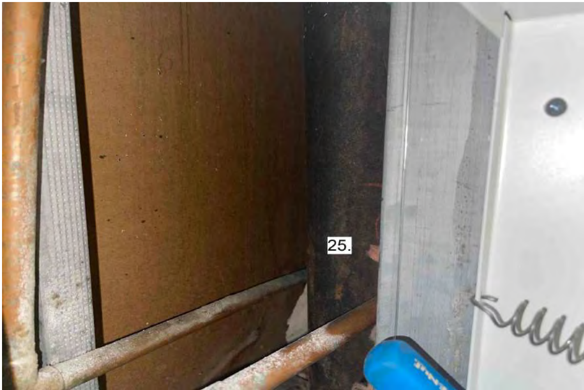
Photograph 13: 12 th Floor Bathroom Stack Unit 1201.
