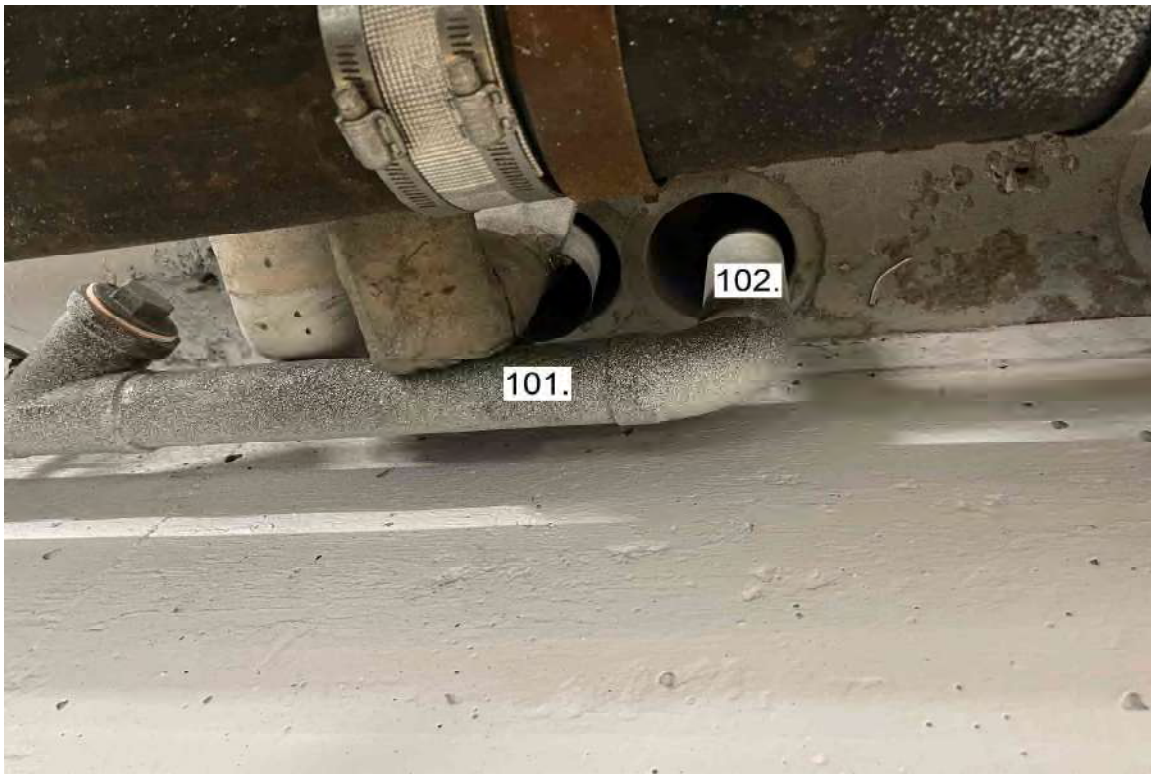
Photograph 29: Public Garage Pillar 9.
