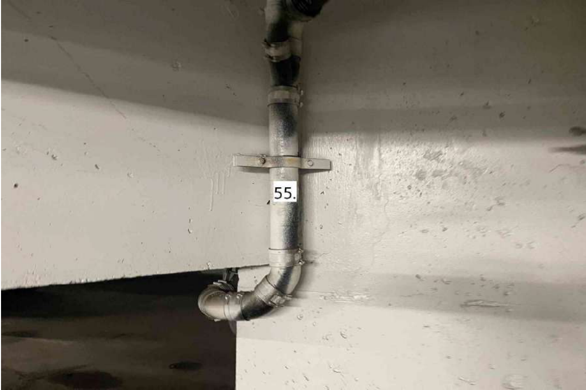
Photograph 16: Condo Garage beside Spot 14.
