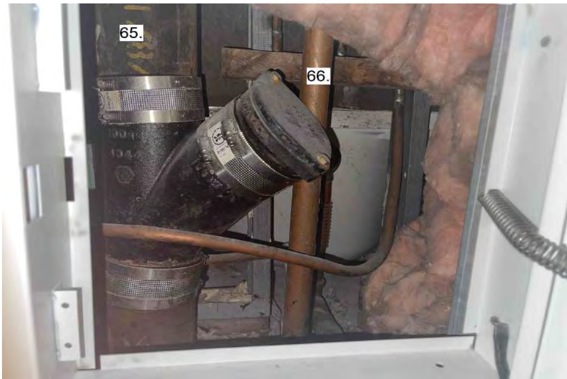
Photograph 34: 4 th Floor Bathroom Stack Unit 406.
