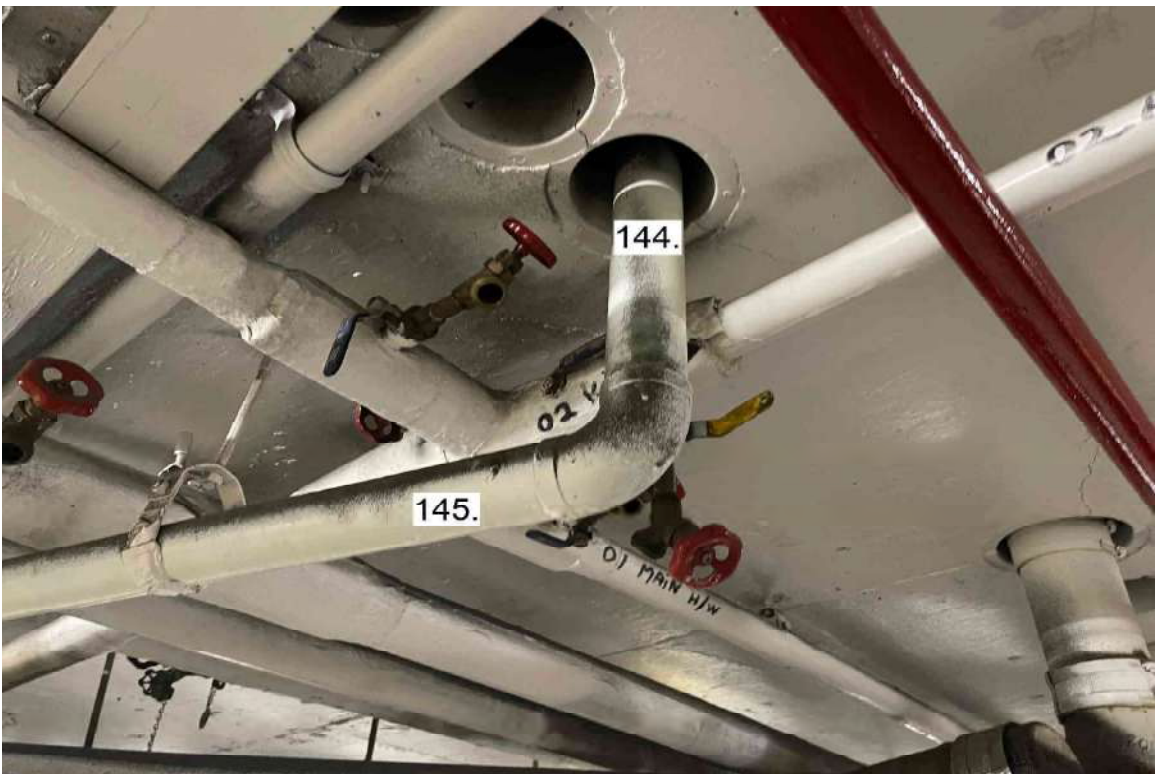
Photograph 44: Level 1 Garage Spot 29.
