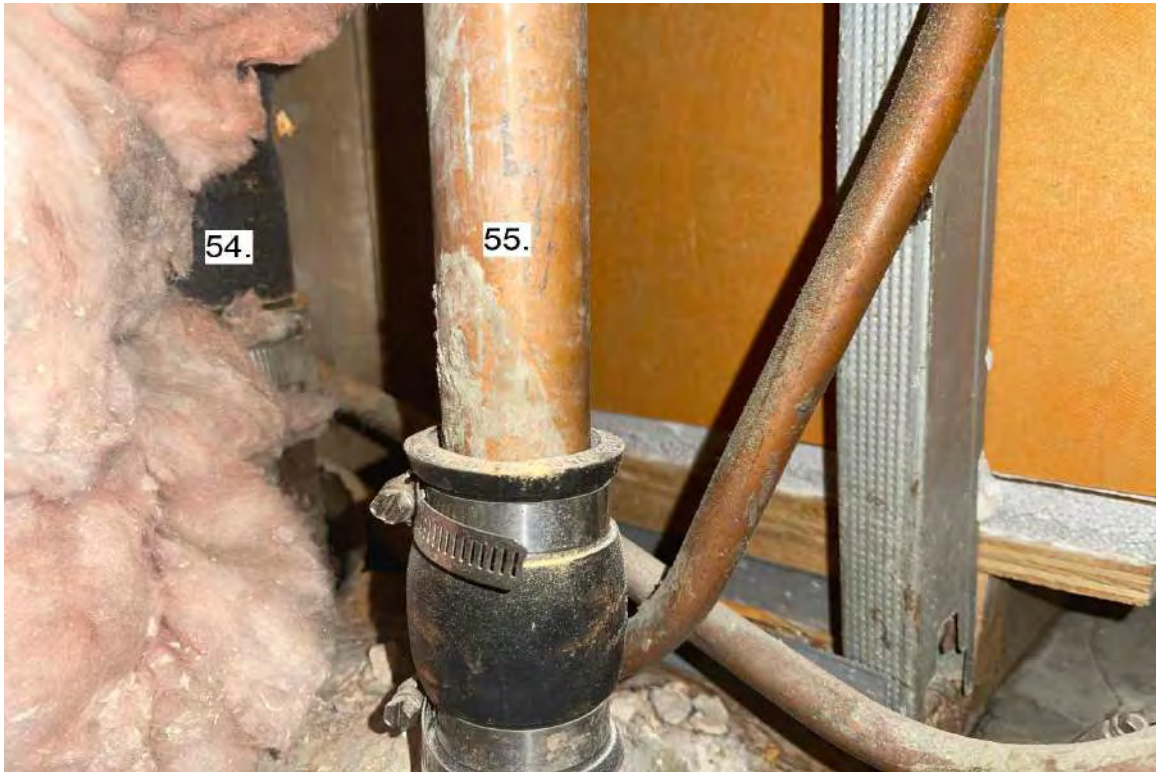
Photograph 29: 5 th Floor Bathroom Stack Unit 510.
