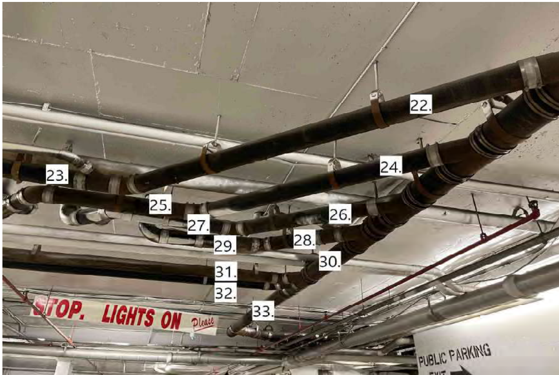
Photograph 7: Between Public Parking & Condo Garage.
