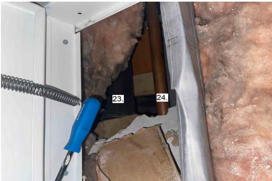
Photograph 12: 14 th Floor Bathroom Stack by 1406.
