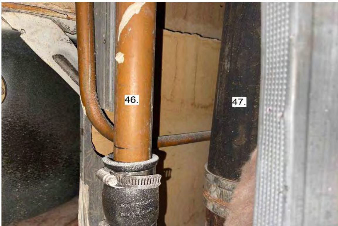
Photograph 24: 6 th Floor Bathroom Stack Unit 602.
