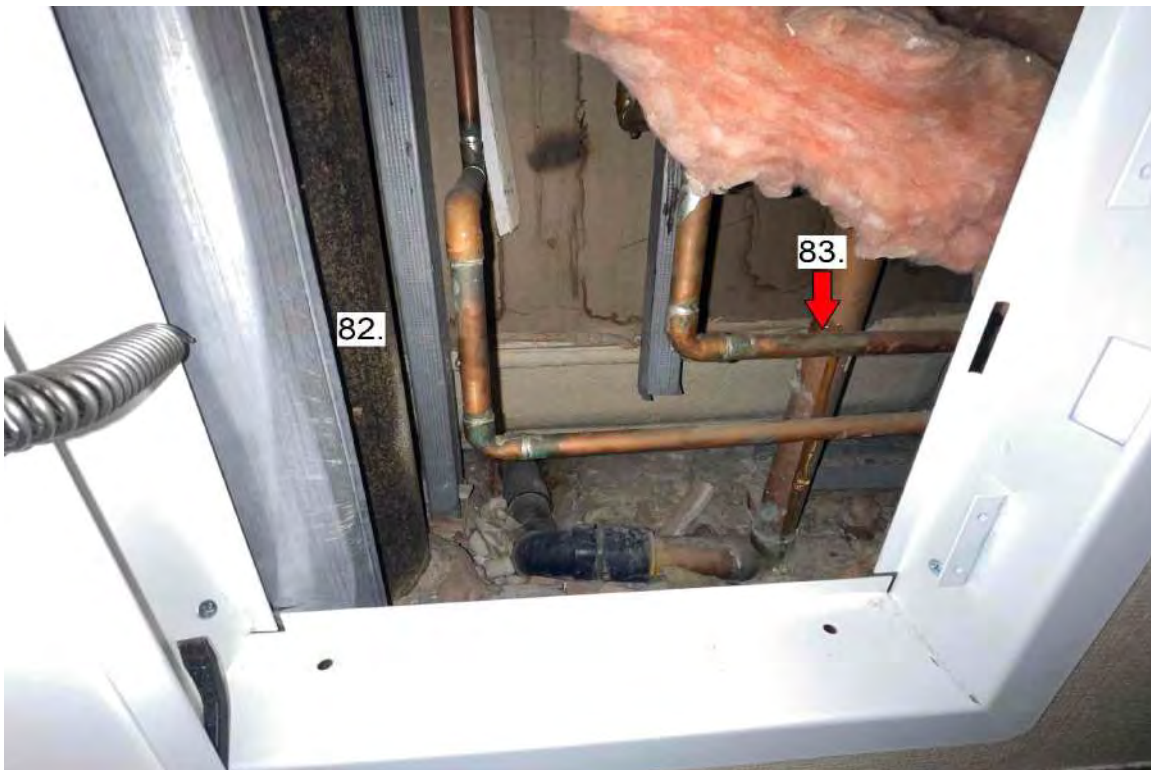
Photograph 44: Ground Level Bathroom Stack Unit 107.
