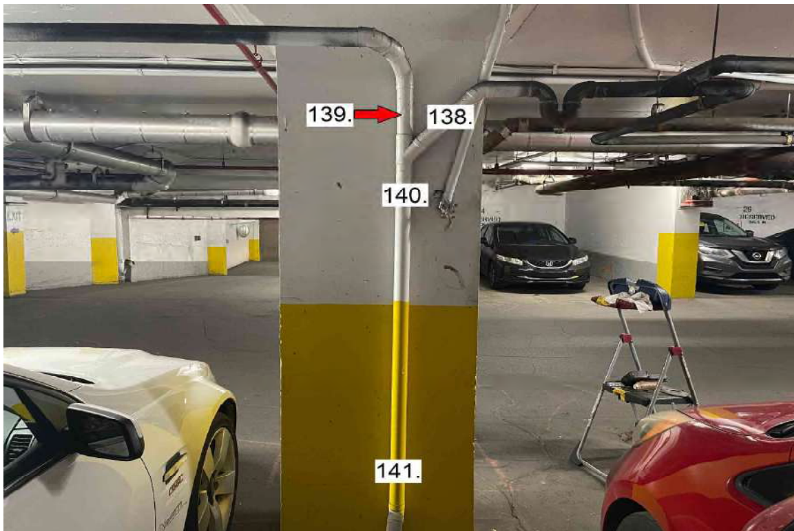
Photograph 42: Level 1 Garage Pillar 21.
