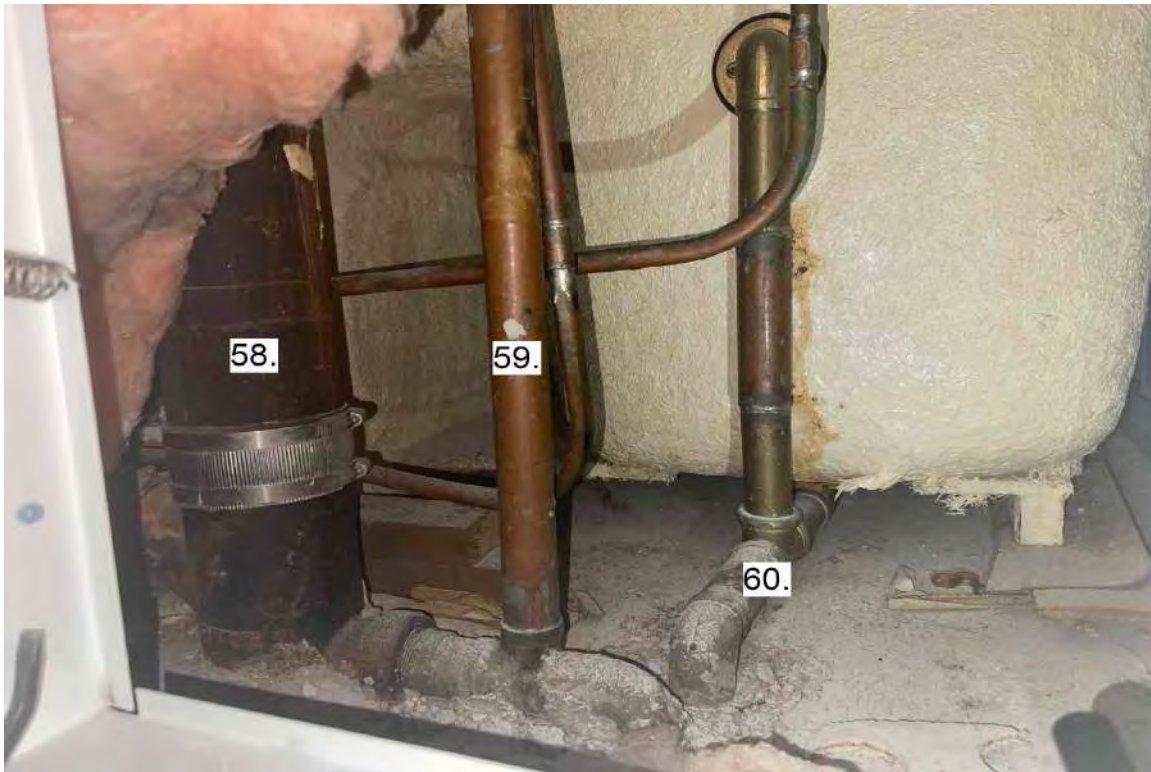
Photograph 31: 5 th Floor Bathroom Stack Unit 506.
