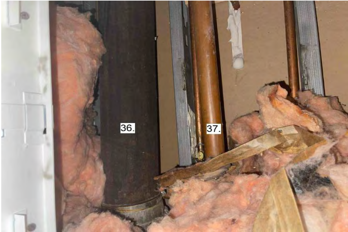
Photograph 19: 8 th Floor Bathroom Stack Unit 806.
