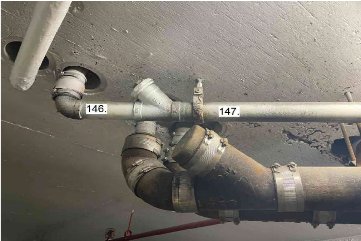
Photograph 45: Level 1 Garage Spot 29.
