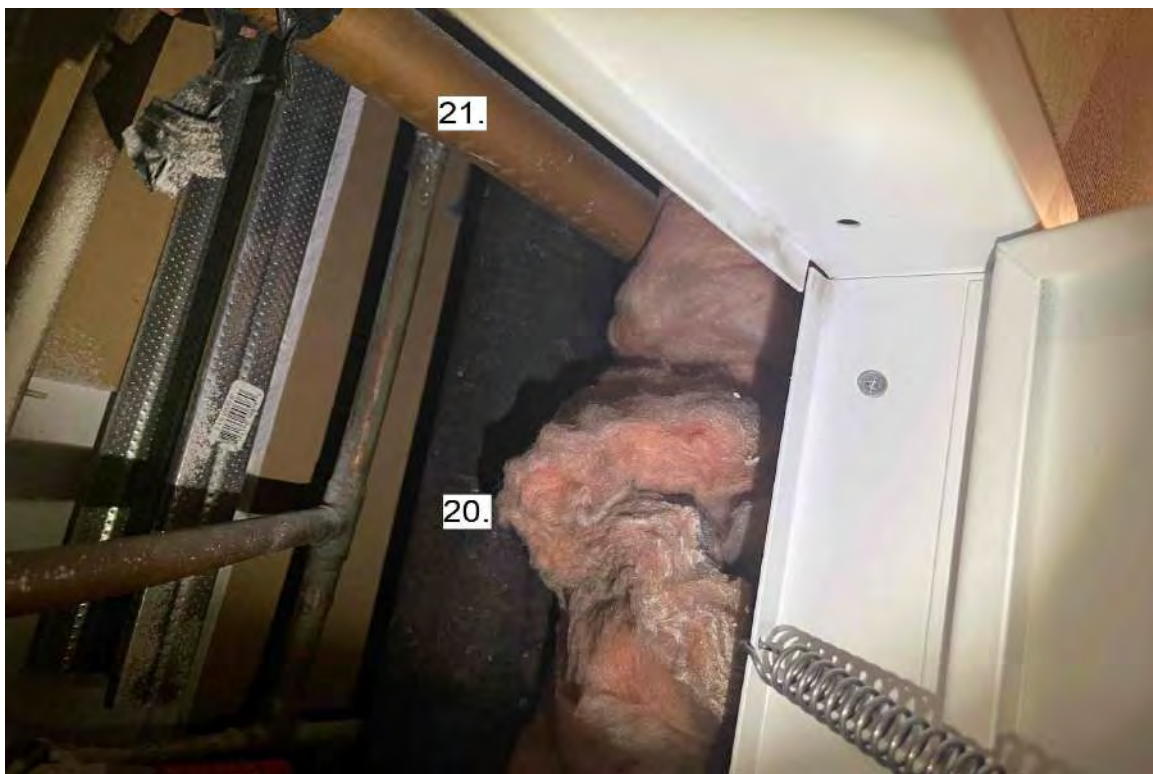
Photograph 10: 14 th Floor By Stairwell 14A.
