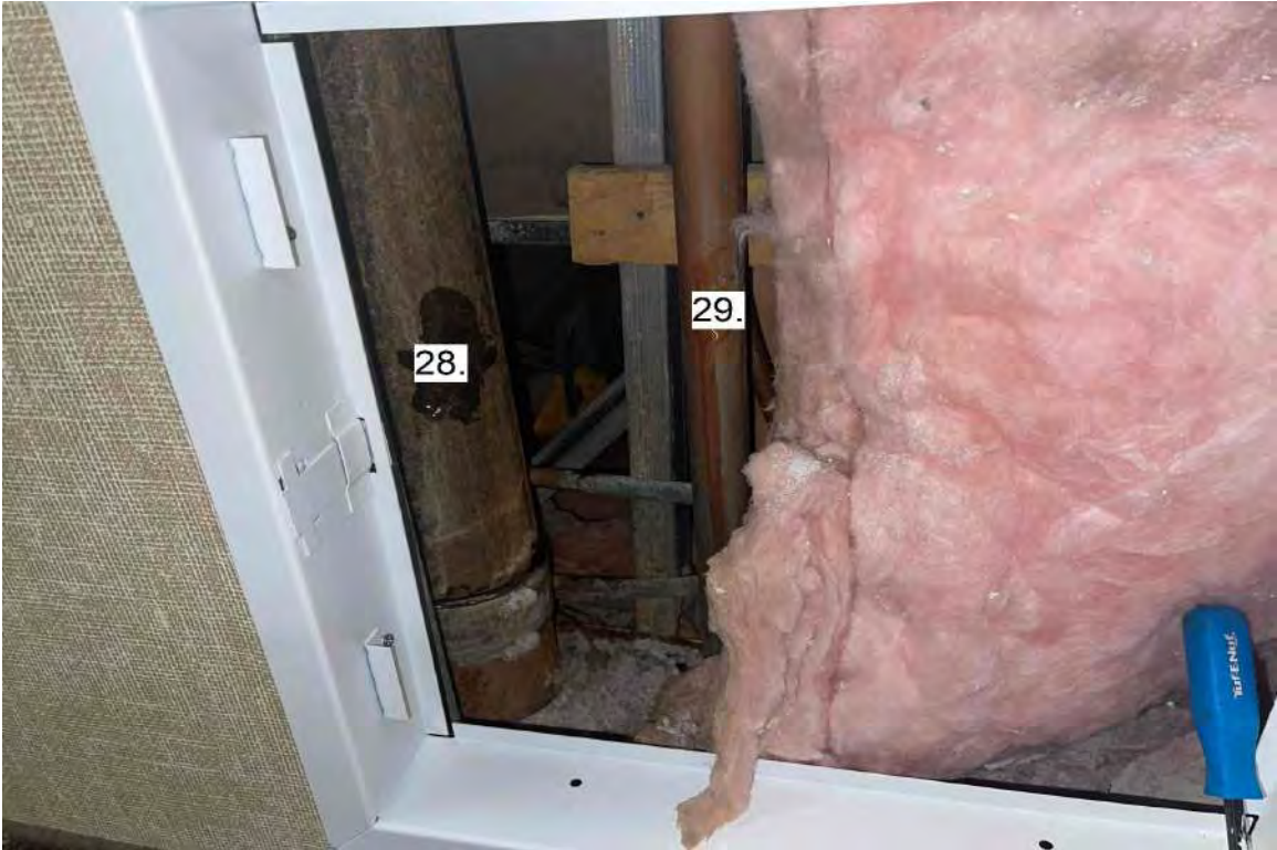
Photograph 15: 10 th Floor Bathroom Stack Unit 1001.
