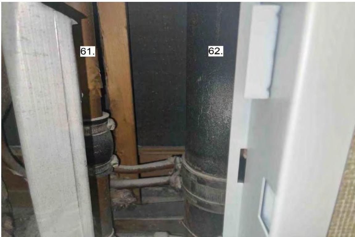
Photograph 32: 5 th Floor Bathroom Stack Unit 502.
