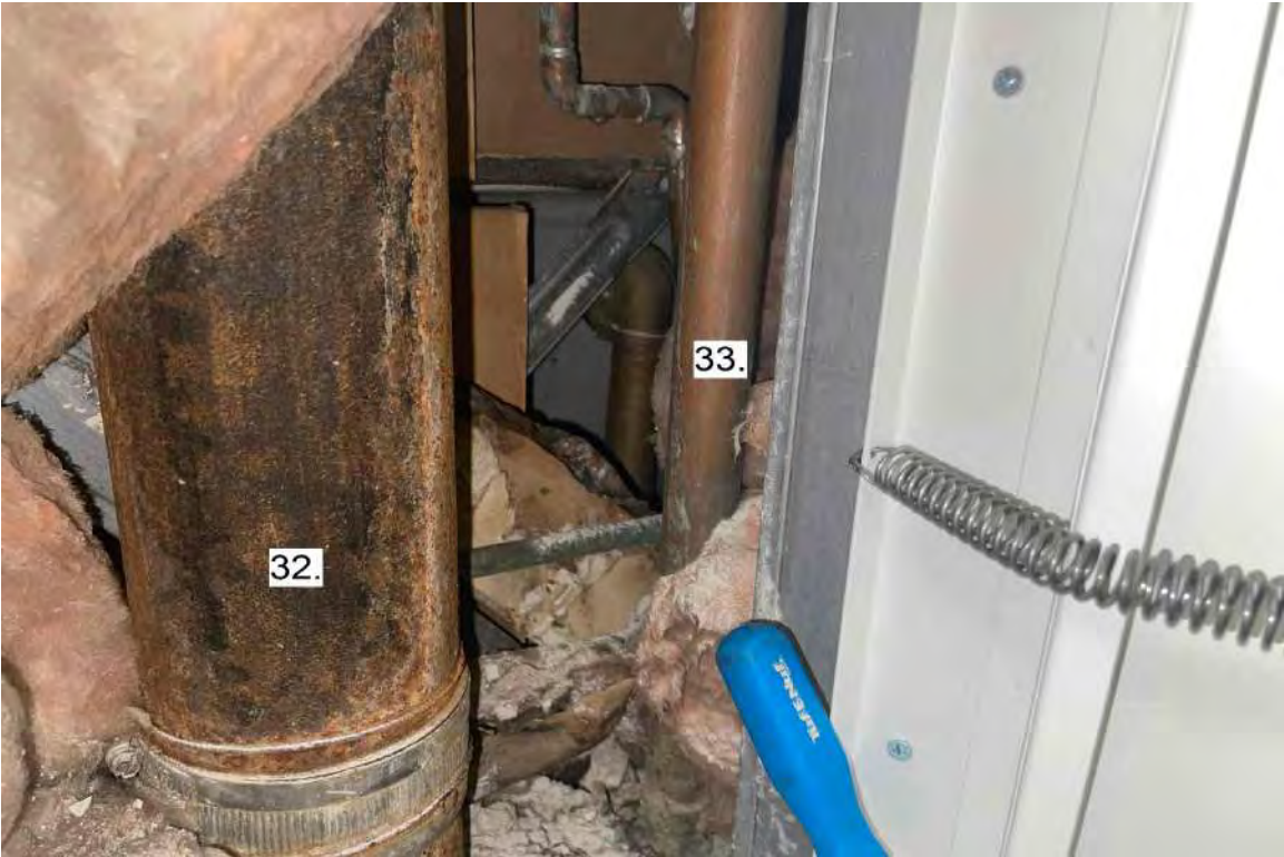
Photograph 17: 9 th Floor Bathroom Stack Unit 901.
