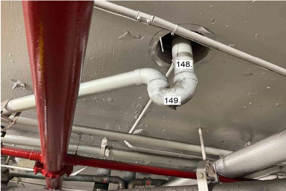
Photograph 46: Level 1 Garage Spot 29.
