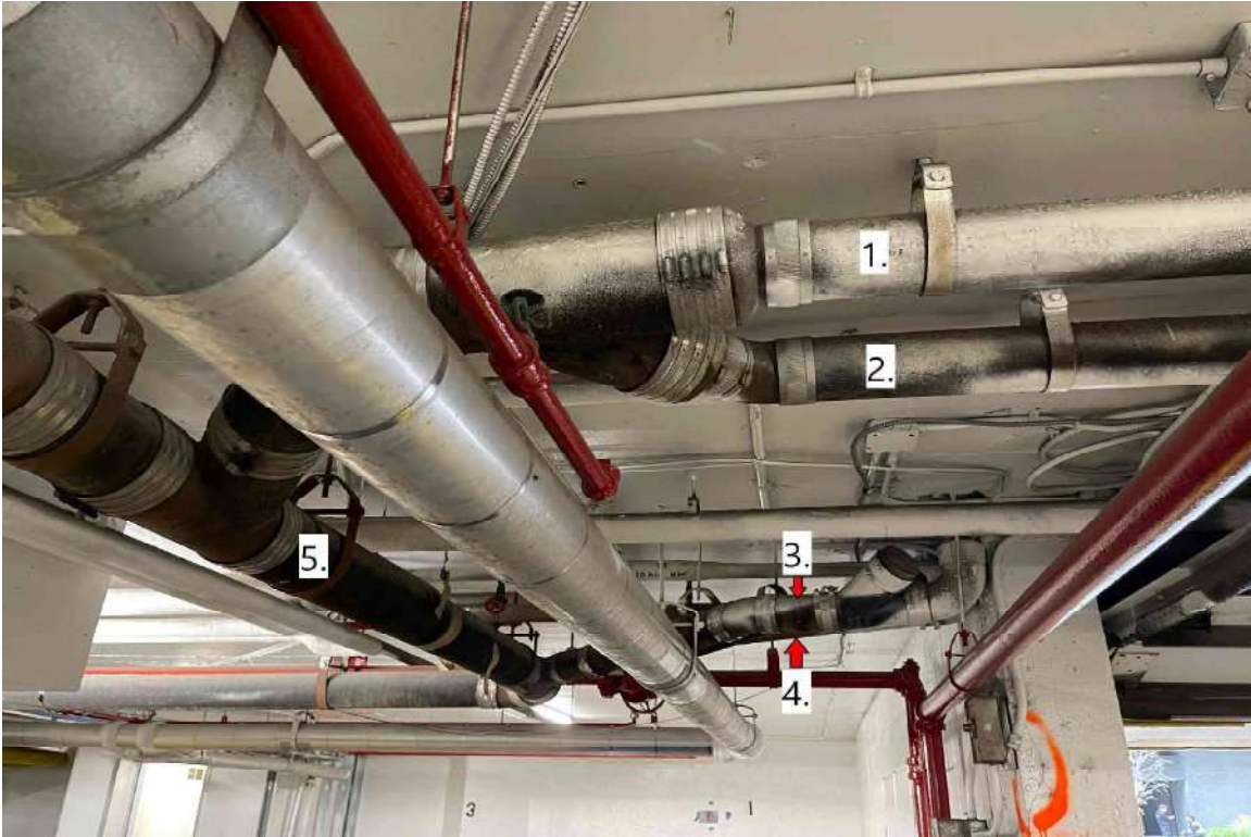
Photograph 1: Parking Garage 1 Entrance.
