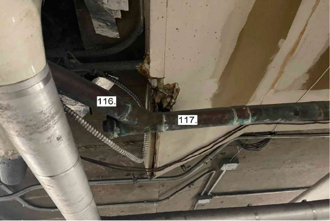
Photograph 34: Building Garage Entrance & Exit.
