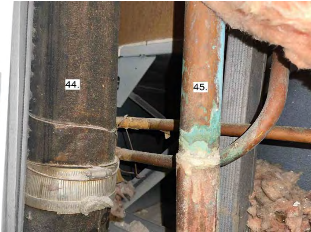
Photograph 23: 7 th Floor Bathroom Stack Unit 707.
