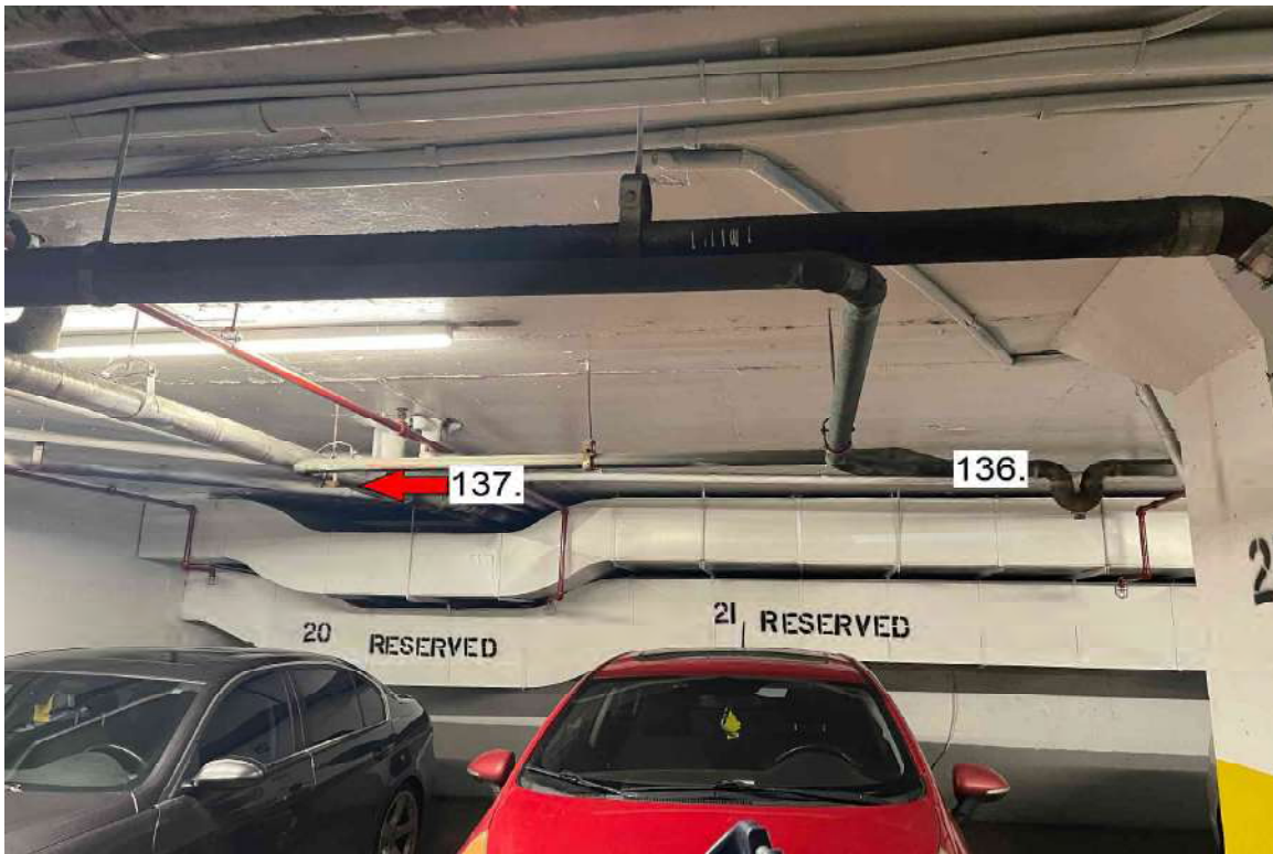
Photograph 41: Level 1 Garage Spot 20 & 21.
