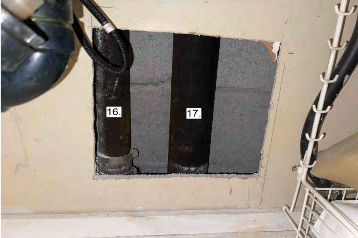
Photograph 8: 2 nd Floor Unit 206.
