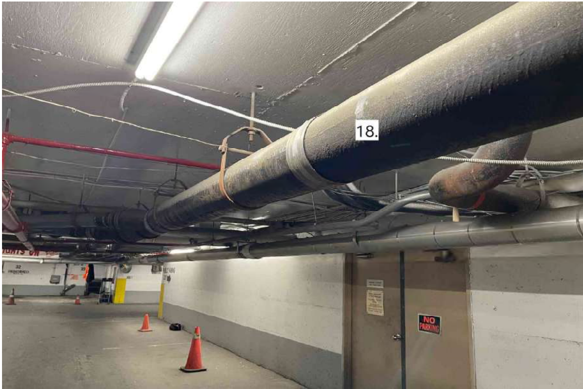
Photograph 5: Between Public Parking & Condo Garage.
