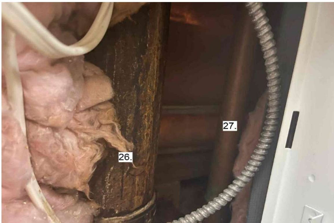
Photograph 14: 11 th Floor Bathroom Stack Unit 1101.
