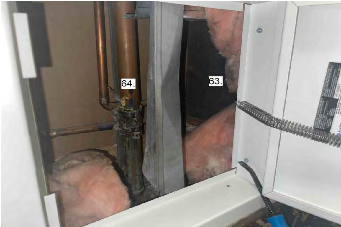
Photograph 33: 4 th Floor Bathroom Stack Unit 402.
