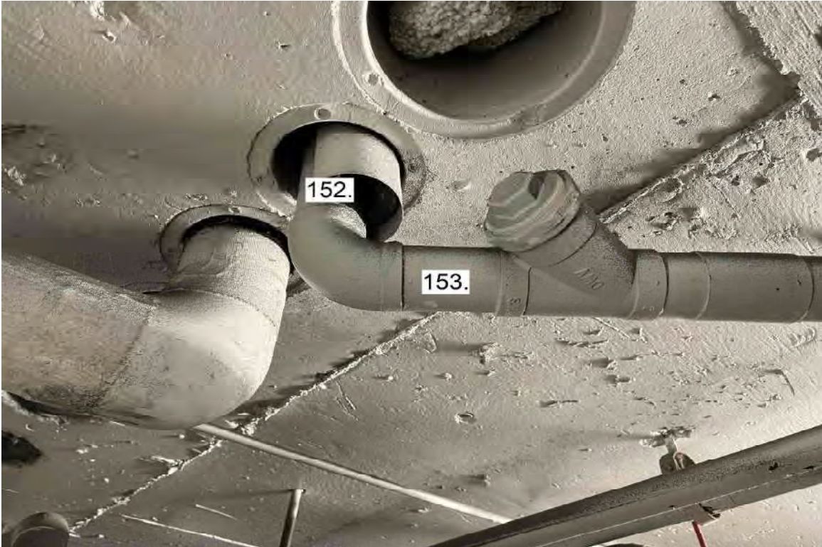
Photograph 48: Level 1 Garage Spot 30.
