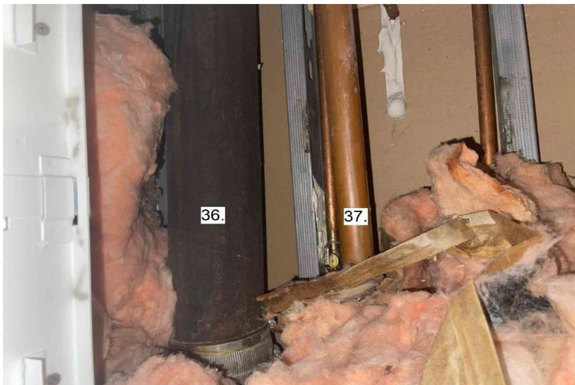
Photograph 19: 8 th Floor Bathroom Stack Unit 806.
