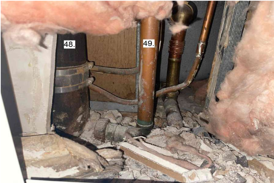
Photograph 25: 6 th Floor Bathroom Stack Unit 606.
