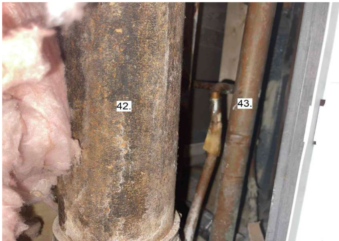
Photograph 22: 7 th Floor Bathroom Stack Unit 701.
